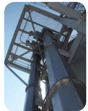
Typical two stage vertical lift sludge conveyors feeding a storage silo
